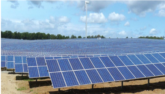
Location: San Floro, Calabria, Italy Project Type: Ground Mounted Project Scale : 24 MWp
