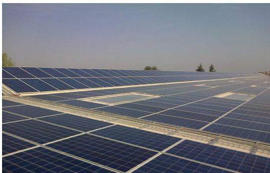
Six Energy Location: Emilia Romagna, Italy Location Type: Roof Top Project Scale: 2,3 MWp
